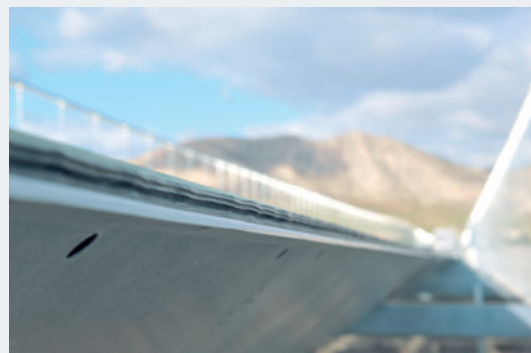
Despite strong sunlight, the Terostat MS adhesive keeps the mirrors fixed to their steel frames.
